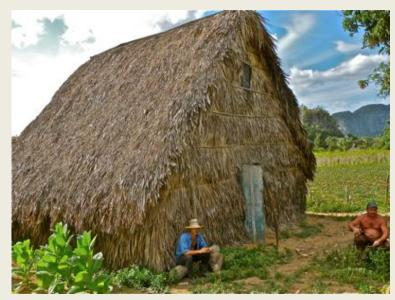
A natural roof is chaeaper but it needs repair every now and then. Of course, bugs feel at home in such houses, too, but it's not as loud inside when it rains and it does not become as hot when the sun is shining. The angle of the roof should be 60 degrees in order to reduce the impact of the water. Otherwise, rain easily passes through the roof.
